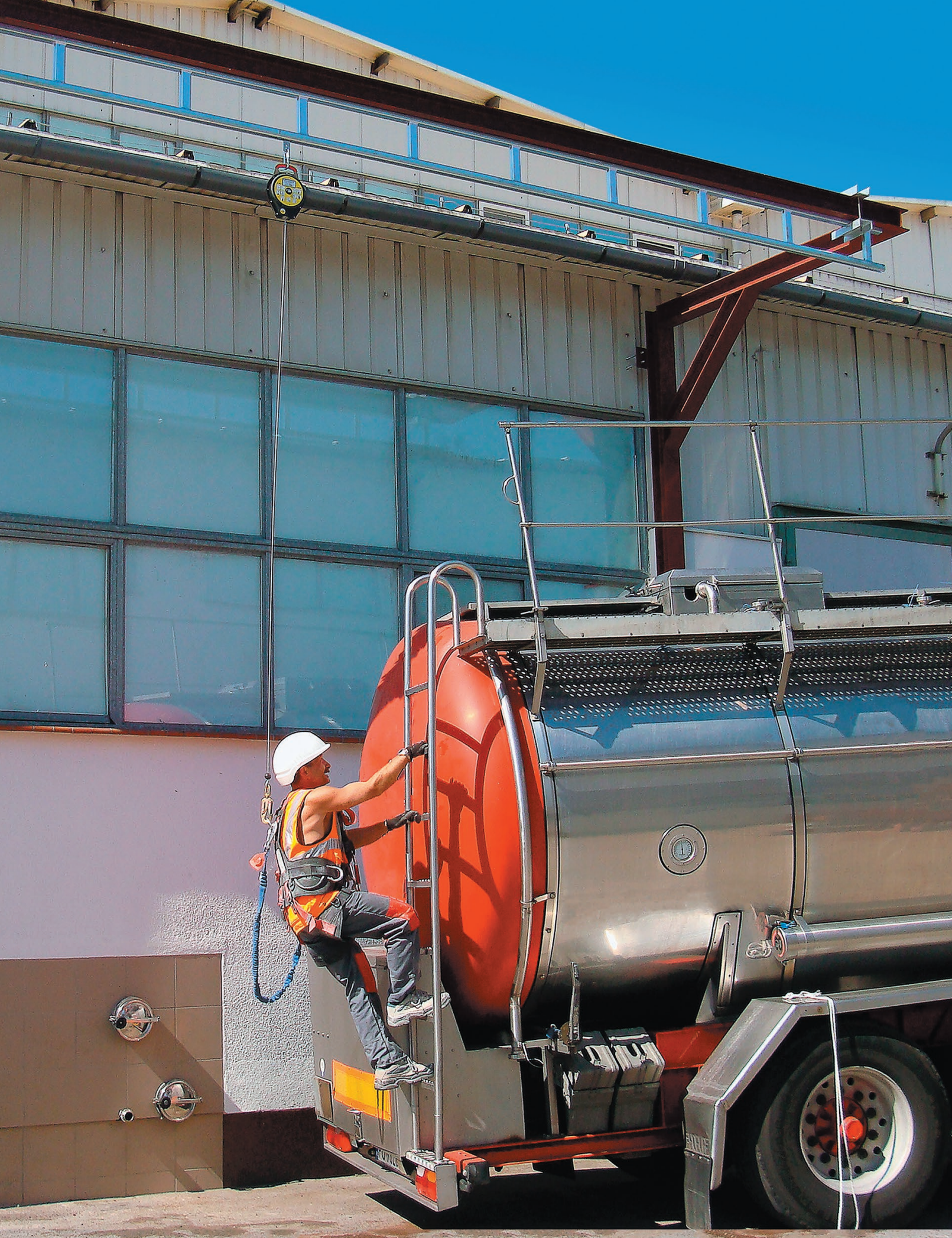
PROTEKT ® Example configuration of TRASER system on a ramp.
